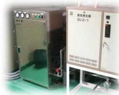
Humidifying water for printing machine
