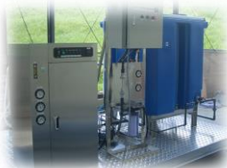
Cleaning water for chiller scale
