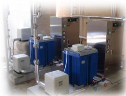
Humidifying water for air conditioner
